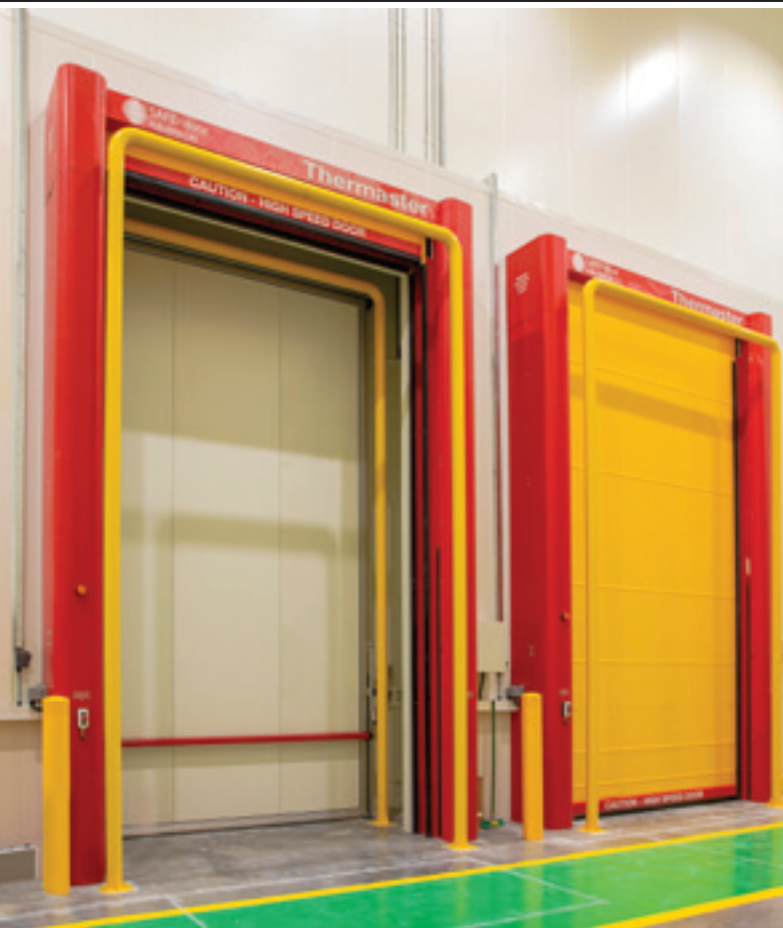
HIGH SPEED DOORS (CHILLER & FREEZER)
